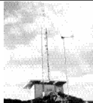
Professional Telecommunications Site Papua New Guinea - 14000ft.
